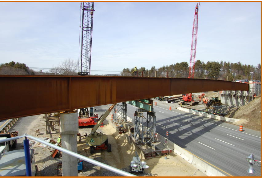
STRUCTURAL STEEL SET ~ APRIL 2008
