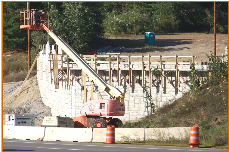
EAST BRIDGE ABUTMENT
