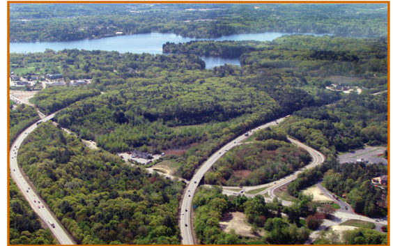
EXIT 3 AREA BEFORE CONSTRUCTION
