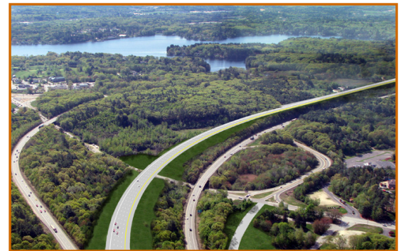
EXIT 3 AREA INTERIM CONSTRUCTION
