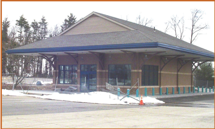
Exit 4 Bus Terminal Nearing Completion March 24, 2007
