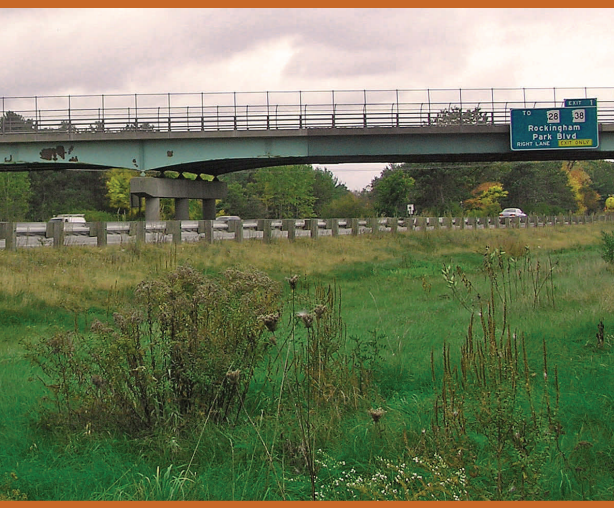
Existing Cross Street Bridge
