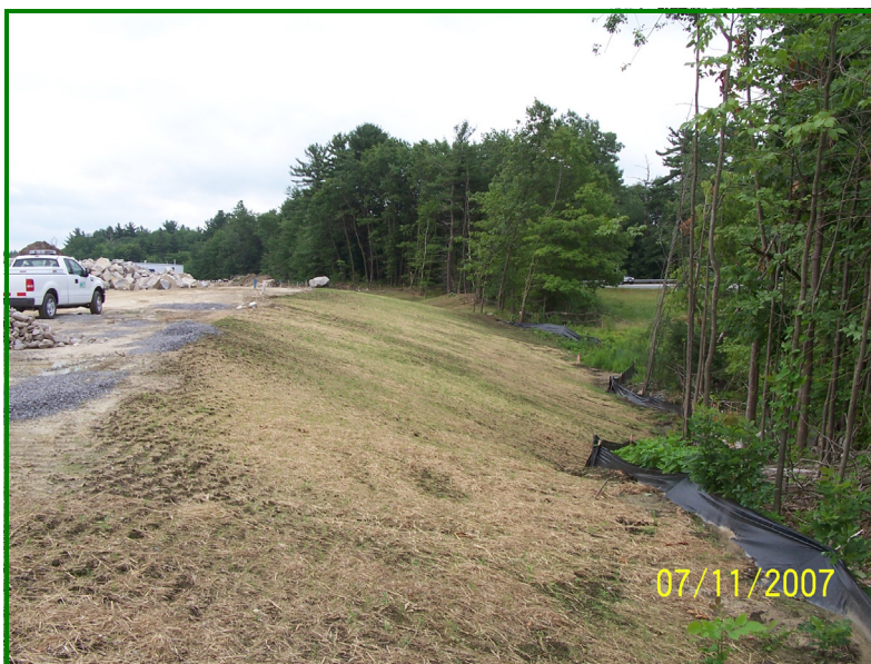
Note turf establishment on slope and placement of silt fence to prevent erosion.
