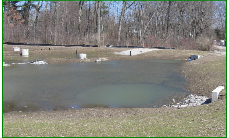
RECENTLY CONSTRUCTED GRAVEL WETLAND DETENTION BASIN AT EXIT 2 PARK-AND-RIDE
