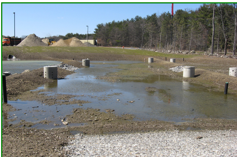
RECENTLY CONSTRUCTED GRAVEL DETENTION WETLAND BASIN AT EXIT 2 PARK-AND-RIDE
