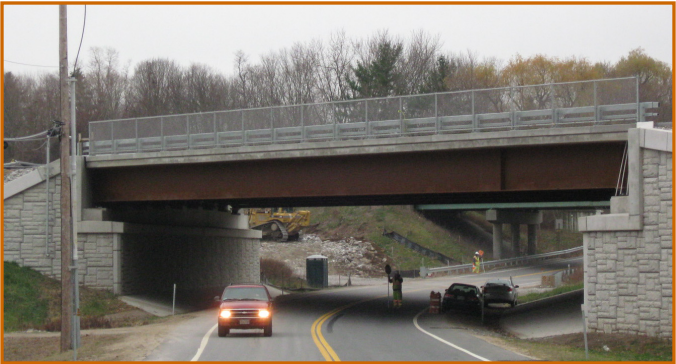
Northbound Bridge over Route 111A
