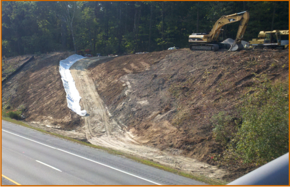
Construction of Temporary Ramp to Staging Area
