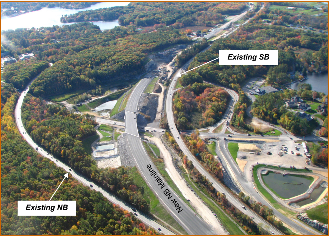
AERIAL VIEW OF NEW SECTION OF NB (LOOKING SOUTH) MAINLINE, INCLUDING NEW BRIDGE OVER ROUTE 111
