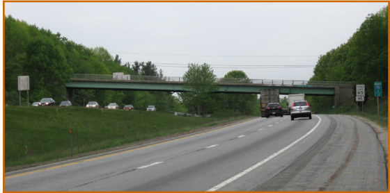
Existing Brookdale Road Bridge
