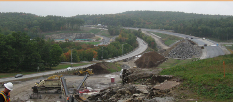
LOOKING NORTH, ROUTE 111 BRIDGE EXISTING SB ON LEFT, NEW NB ON RIGHT
