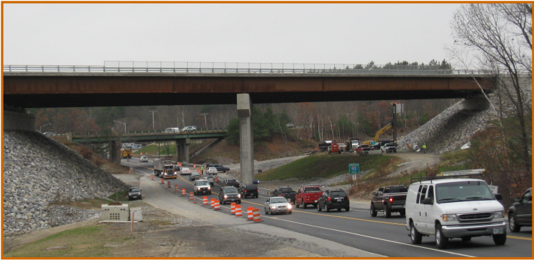
Northbound Bridge over Route 111
