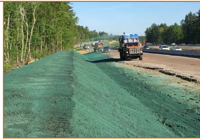
LEFT: I-93 SB soundwall berm hydroseeding, facing north. ABOVE: Workers tying rebar intersections on SB Bridge over Stonehenge Road approach slab, facing north.
