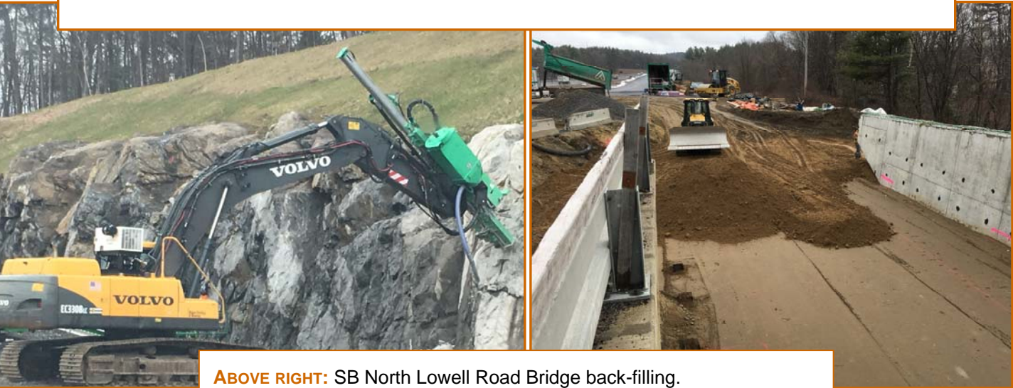
ABOVE RIGHT: SB North Lowell Road Bridge back-filling. ABOVE LEFT: Installation of rock bolts and dowels in southern ledge cut.
