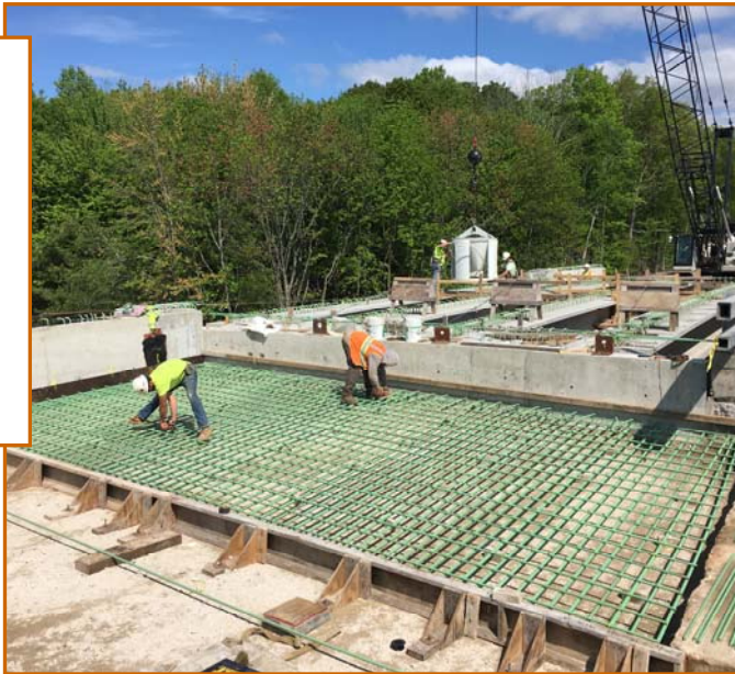
LEFT: I-93 SB soundwall berm hydroseeding, facing north. ABOVE: Workers tying rebar intersections on SB Bridge over Stonehenge Road approach slab, facing north.
