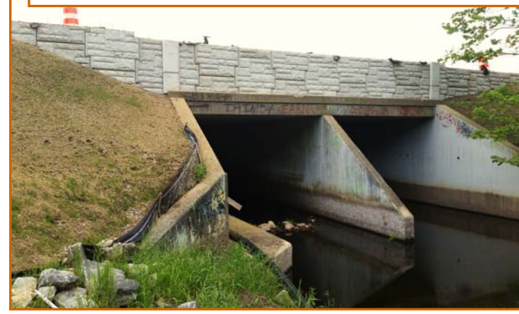
LEFT: The last of the MSE wall panels were installed at the northern box culvert. RIGHT: Paving.
