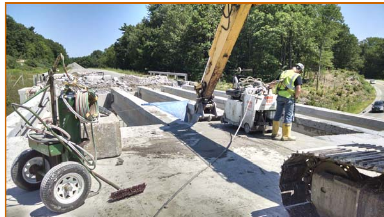
Removal of bridge deck from old NB over NH 111A
