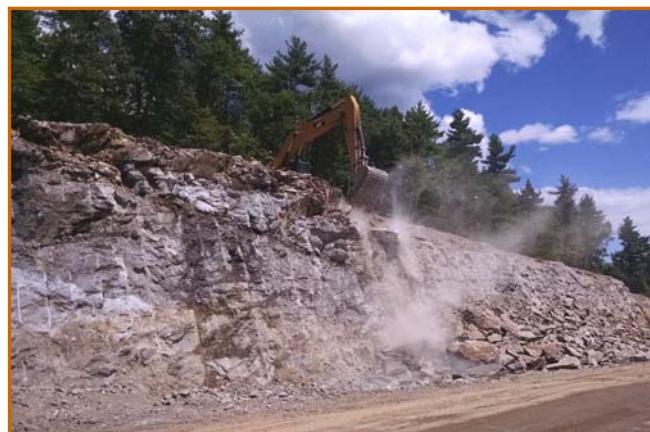
Clearing of loose rock from ledge cut
