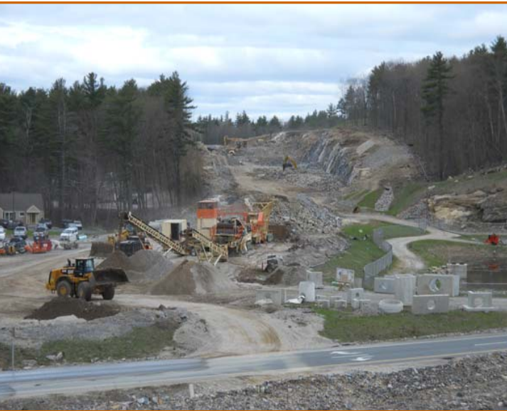
Rock cut/earth work for relocation of Route 111 west of I-93 (Looking West)
