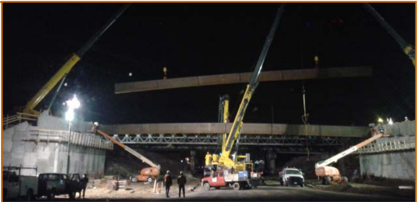
Setting Steel for new SB Bridge
