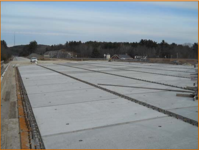
SB Bridge over Route 111A, with Deck Panels Installed
