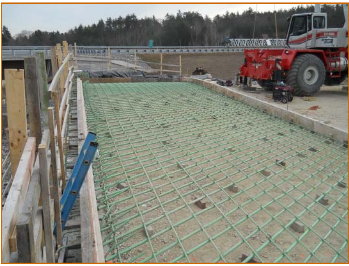
SB Bridge over Route 111A, Slab Steel Reinforcement December 2012 - 70% Complete
