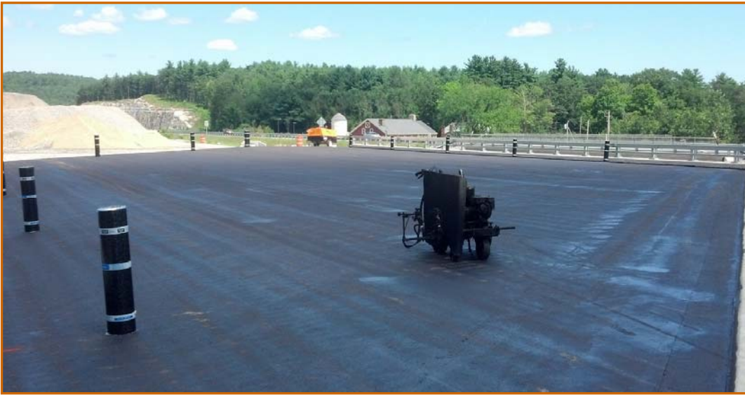
Route 111A Deck with Rail and Primer 08-13
