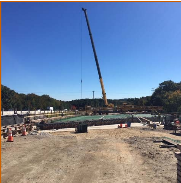
SB NORTH LOWELL ROAD BRIDGE
