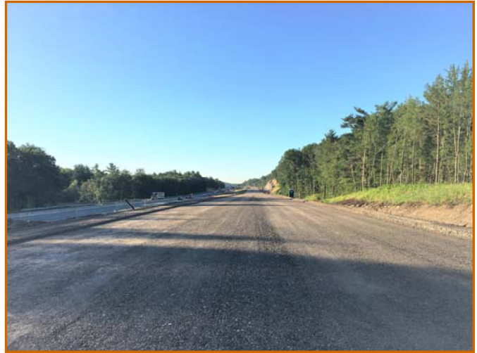
FINE GRADING OF SB ROADWAY SELECTS
