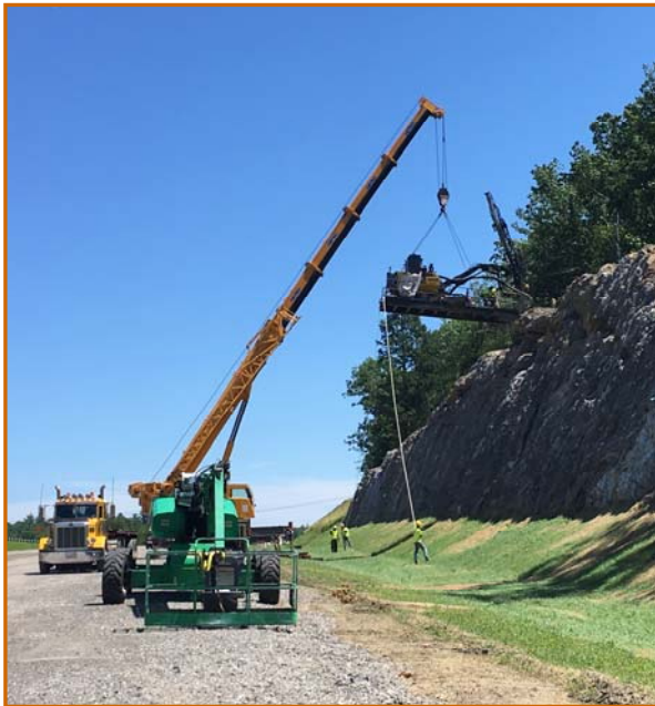
ROCK BOLT INSTALLATION ON SB LEDGE CUT
