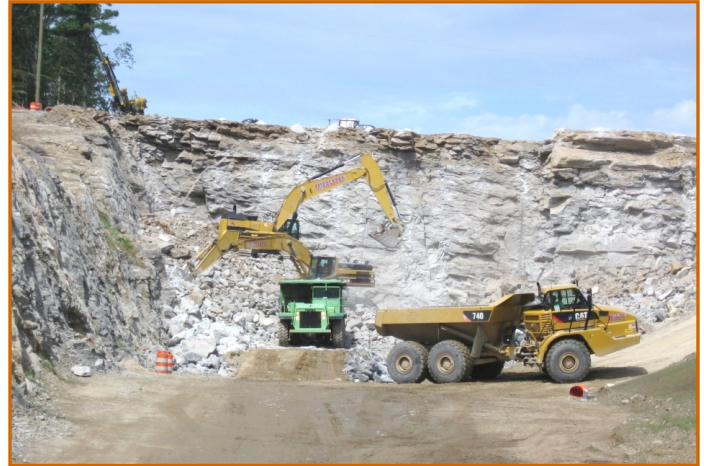
BLASTING & LEDGE/ROCK REMOVAL OPERATIONS
