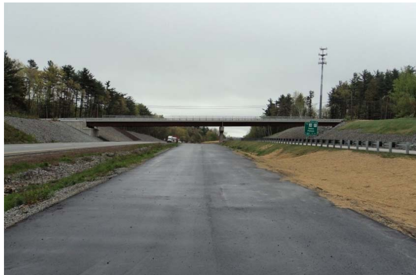
LOOKING SOUTH AT NEW BROOKDALE ROAD BRIDGE, 05-03-2012
