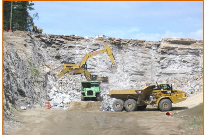
BLASTING & LEDGE/ROCK REMOVAL OPERATIONS
