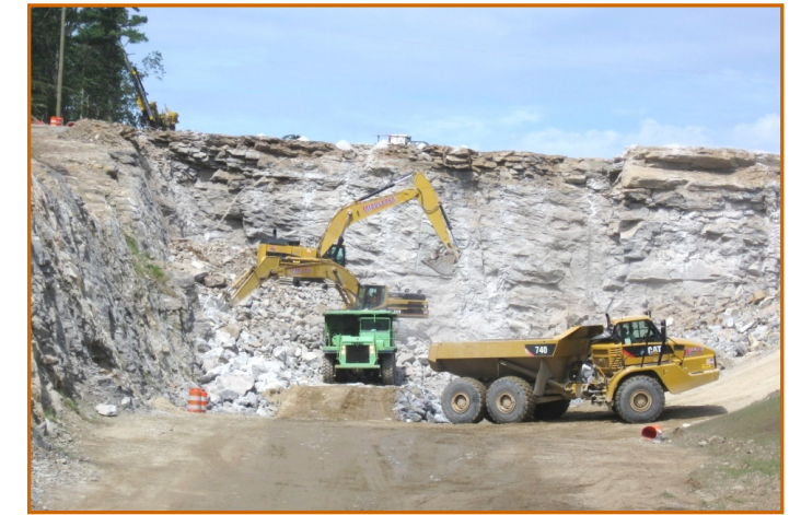
ROCK & LEDGE REMOVAL OPERATIONS
