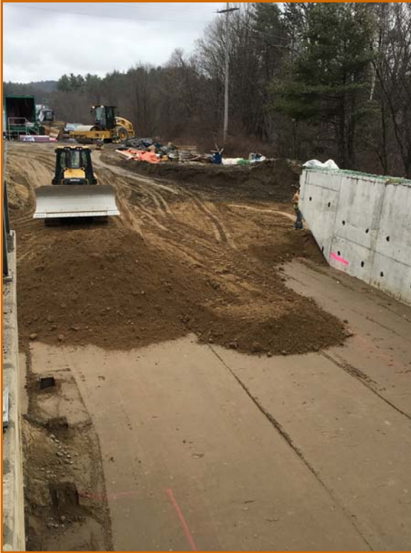
ABOVE: SB NORTH LOWELL ROAD BRIDGE BACK-FILLING
