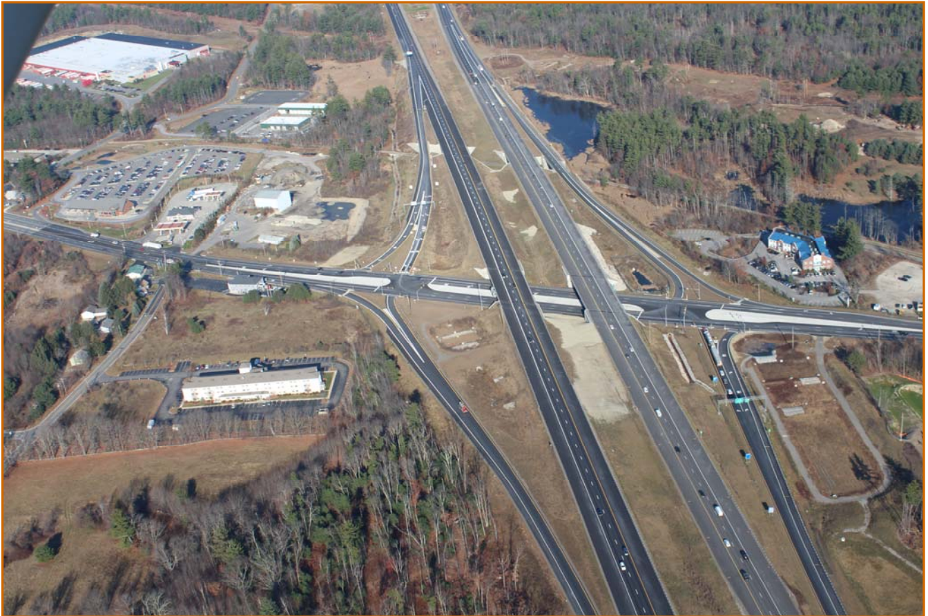
Aerial Photo of Completed Exit 5 Interchange
