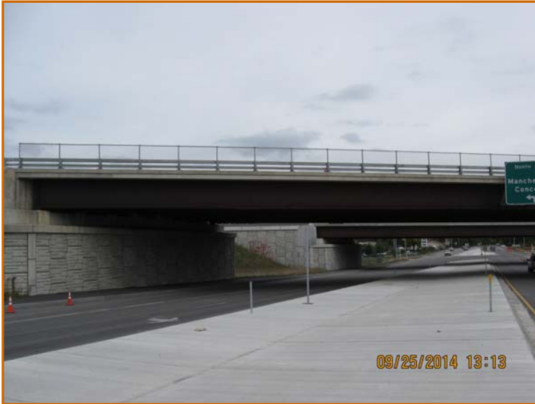
Route 28 improvements under new I-93 bridges
