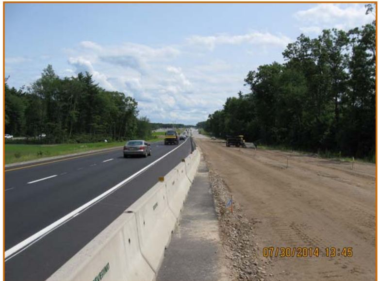
Subbase grading prior to Final Paving
